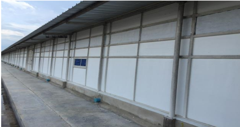
Figure 2. The natural lighting control house
